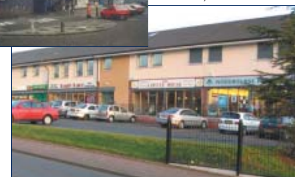
Below - The new SRRP building as it looks today.
