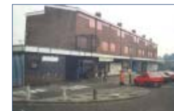
Inset left - Stewartstown Road frontage before demolition, circa 2000.
