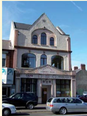
Ballynaveigh Community House. Photo: Ballynaveigh Community Development Association (BCDA)
