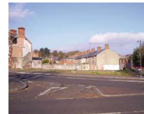
Junction between Glandore & Skegoneil Avenue. These homes have been redeveloped several times but have constantly been vandalised to the extent they are now a health and safety risk. Photo: Malachy Mulgrew
