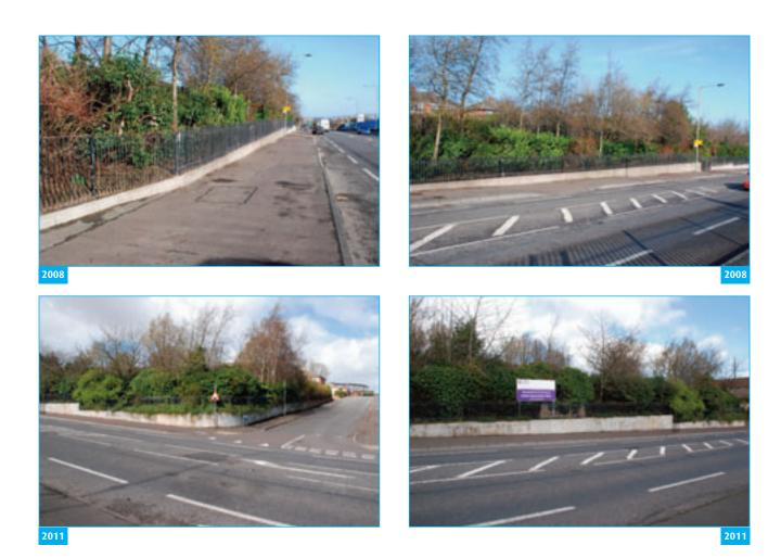
**15. Springfield Parade - West Circular Road (Owner: DoJ. Built: 1980s):** A 2 metre high brick wall with 4 metre high fencing above runs at the rear of properties on the West Circular Road; the barrier then turns 90 degrees and continues as a 2.1 metre high solid metal fence along the face of Springfield Parade.
