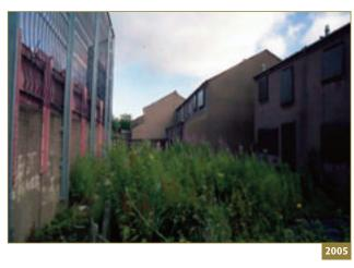
**90. Bryson Street (Owner: DoJ, NIHE maintained. Built: 1970s & 2003):** A brick wall with mesh fencing above, to a total height of 7.5 metres, runs 275 metres along the length of Bryson Street from the junction of Lower Newtownards Road to Madrid Street.
