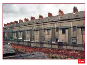
**61. Parkside Gardens (Owner: DoJ. Built: 1995)** A 3.2 metre high mesh fence with 1.2 metre cantilever section atop runs for 70 metres above backyard wall to the terrace of houses on Parkside Gardens. The houses on Mountcollyer Street, on the other side of the fence, have recently been demolished.
