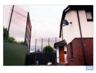
**84. Serpentine Gardens - Gunnell Hill (Owner: DoJ. Built: 1999):** A 3 metre high cladding fence with 6 metre high mesh fencing above runs for 206 metres from Gunnell Hill to Serpentine Road at the rear of properties in Serpentine Gardens.
