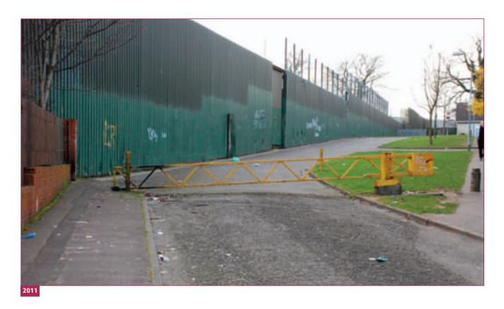
**66. Brucevale Park - Duncairn Avenue (Owner: DoJ. Built: 1978):** A pair of low-level, double swing arm, steel security gates closes off access between these two streets, which run along the boundary of the former Girdwood barracks.
