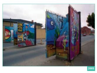
**23. Lanark Way (Owner: DoJ. Built: 1988):** Electronically controlled metal gates, 4 metres high and 10 metres wide, across Lanark Way, between Springfield Road and Merkland Place, can be closed to prevent access.
